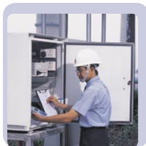
HEC environmental staff calibrating continuous noise monitoring equipment at Lamma Power Station.
